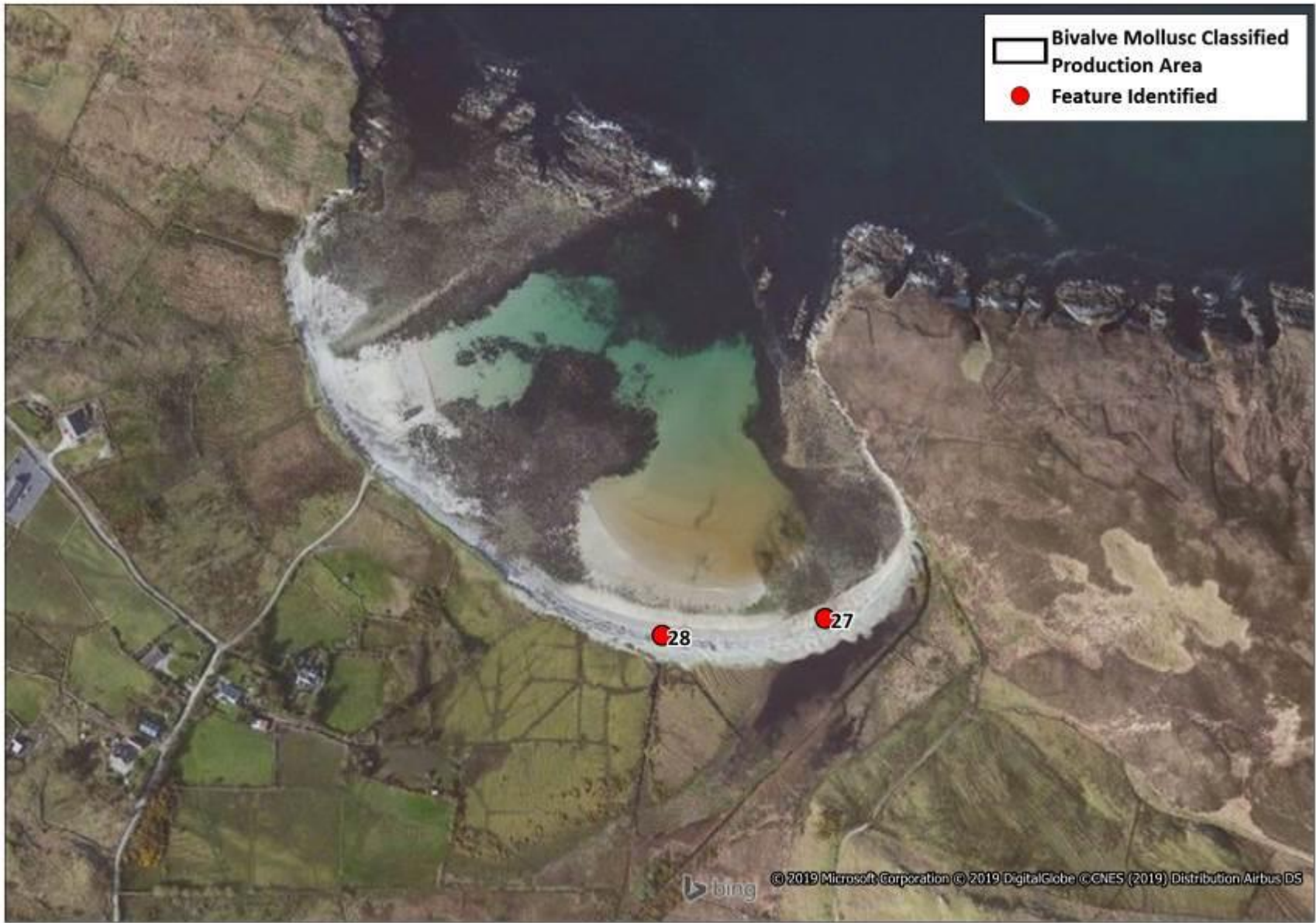
Figure 4.26: Features 27-28 (numbering cross-reference to Table 4.11) identified during the shoreline survey
