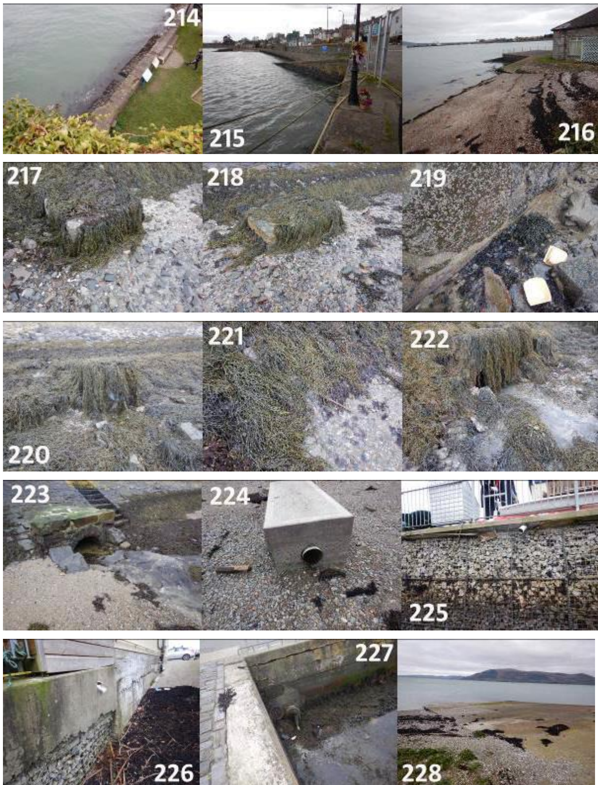
Figure 4.122: Images of features identified in shoreline survey 122-122 (numbering refers to Table 4.8).
