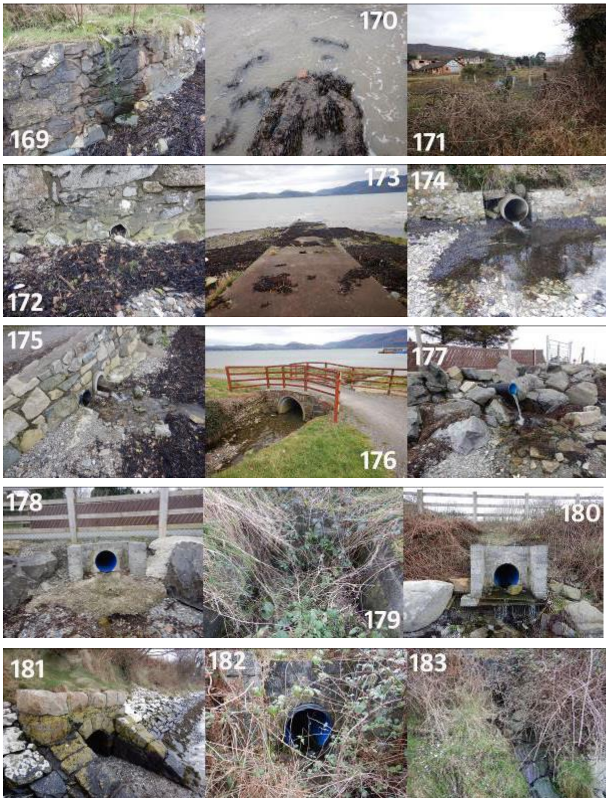
Figure 4.64: Images of features identified in shoreline survey 169-183 (numbering refers to Table 4.8).
