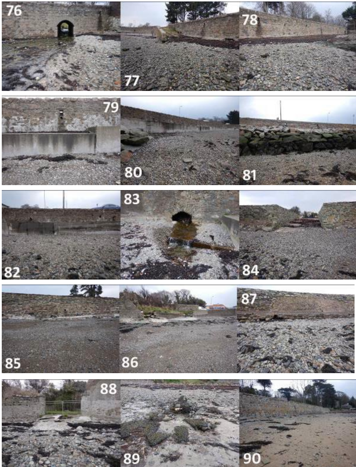
Figure 4.113: Images of features identified in shoreline survey 113-113
