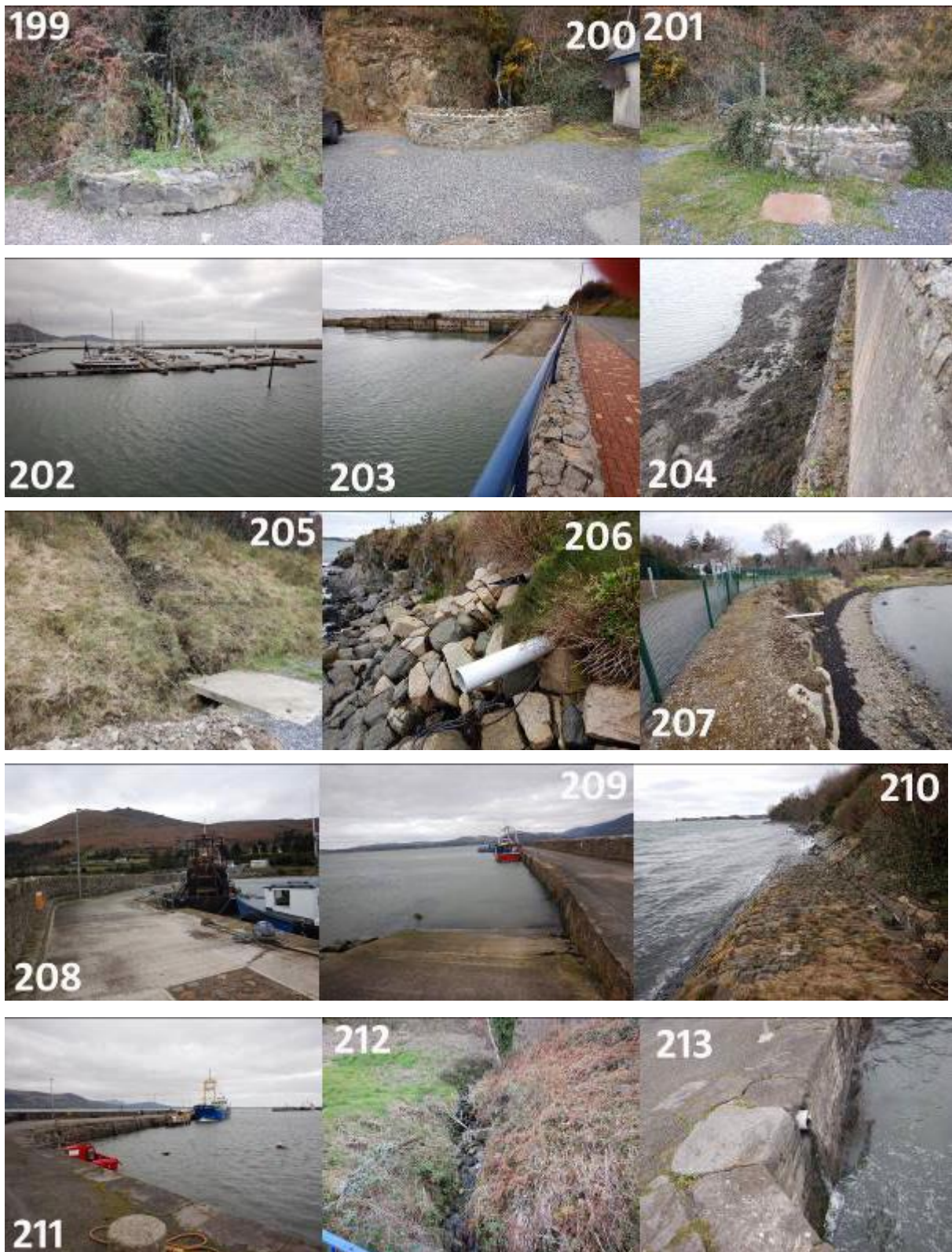
Figure 4.121: Images of features identified in shoreline survey 199-213
