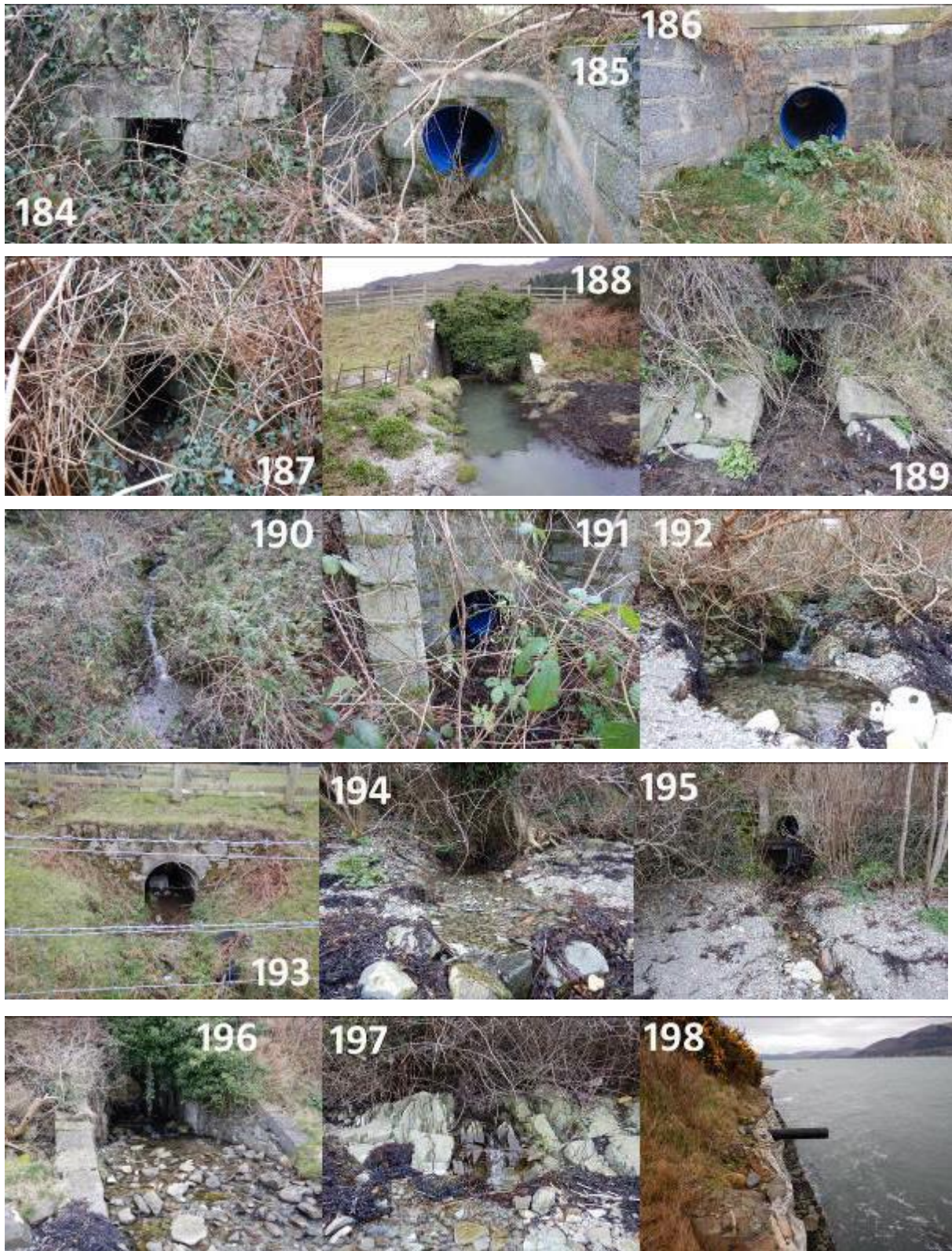
Figure 4.120: Images of features identified in shoreline survey 184-198
